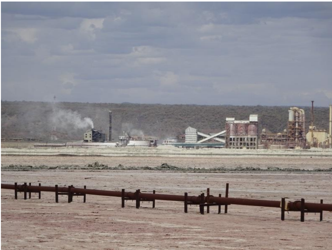
Photo The soda ash factory of TCM in Magadi, and the pipeline bringing in water from Oliborototo.
