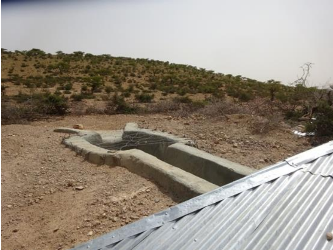
Photo The inlet of a rehabilitated 'berkad' water reservoir in Hareed village, Somaliland.
