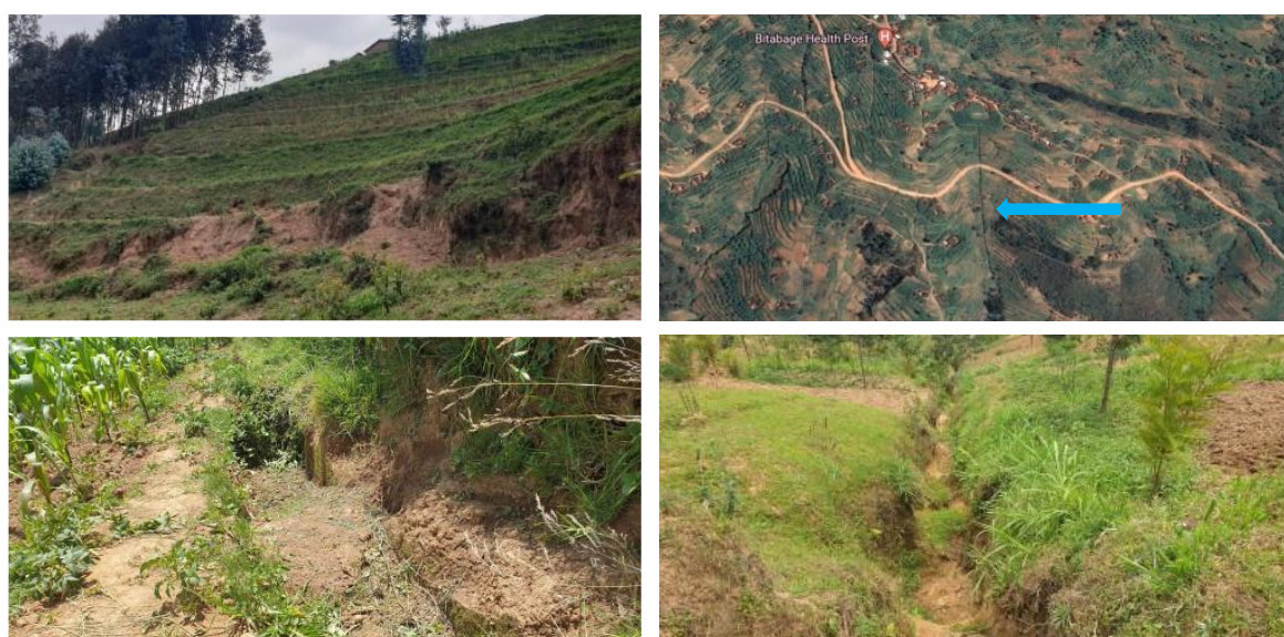
Figure 4 On a limited, case-by-case basis, landscape restoration shows certain limitations. Radical terraces can break and caused localized erosion (top-left); trenches along the contour lines of progressive terraces collect runoff and sediment and eventually break; drains on radical terraces, when not built according to design standards can cause gully erosion downstream (bottom-right).
