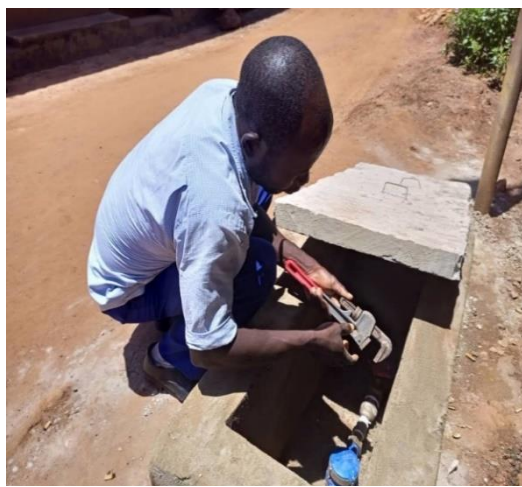
Photo: Akuei Malang Carrying out Plumbing
